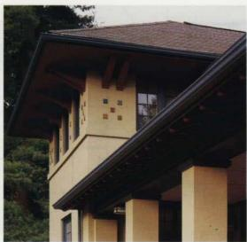
The building's porch (opposite) was rebuilt to include an accessible ramp (far left). Ceramic tiles like those envisioned by the original architects were added under the eaves (left). In the waiting room, paint was removed from wood brackets and the fireplace (below).
